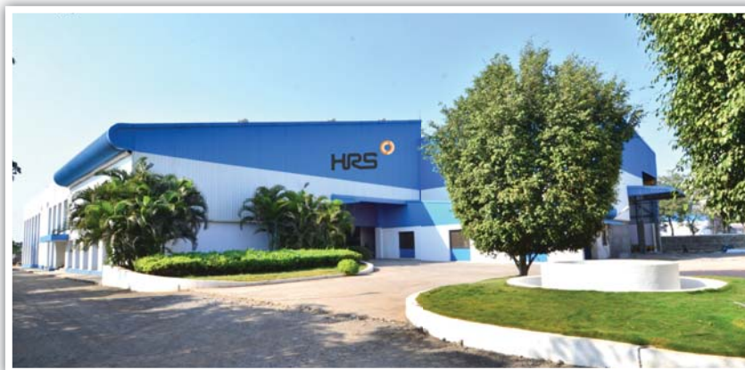
HRS Factory Overview
